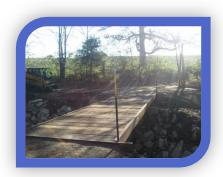
Perimeter Trail Bridge – In fall of 2012, staff built a pedestrian bridge across a creek on the northeast section of the perimeter trail at Big Hollow. The bridge is 30' long, 8' wide, and built almost entirely from old steel and bridge plank from past projects. The bridge allows for the entire perimeter trail to be off of public roads and inside the boundary of the park.
